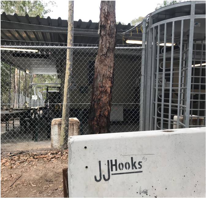
NorthConnex Leased Area
