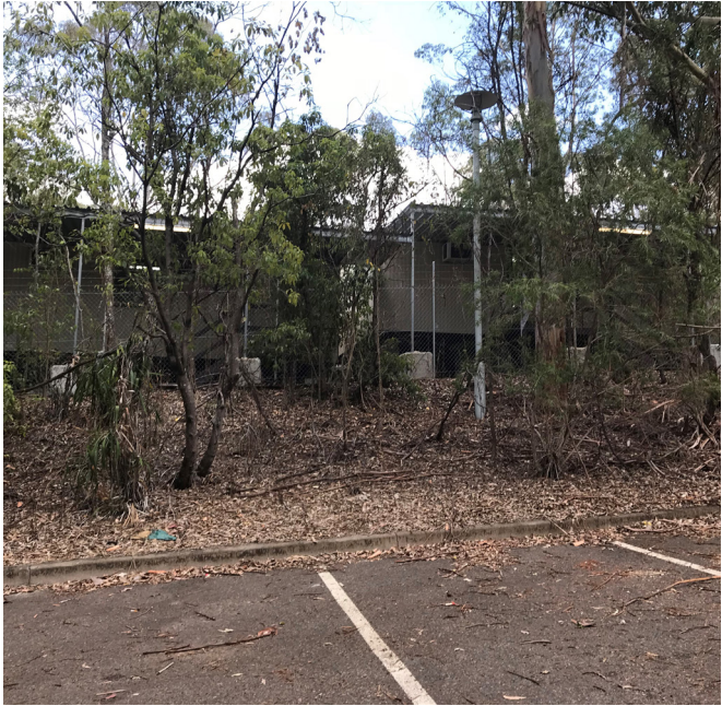
NorthConnex Leased Area
