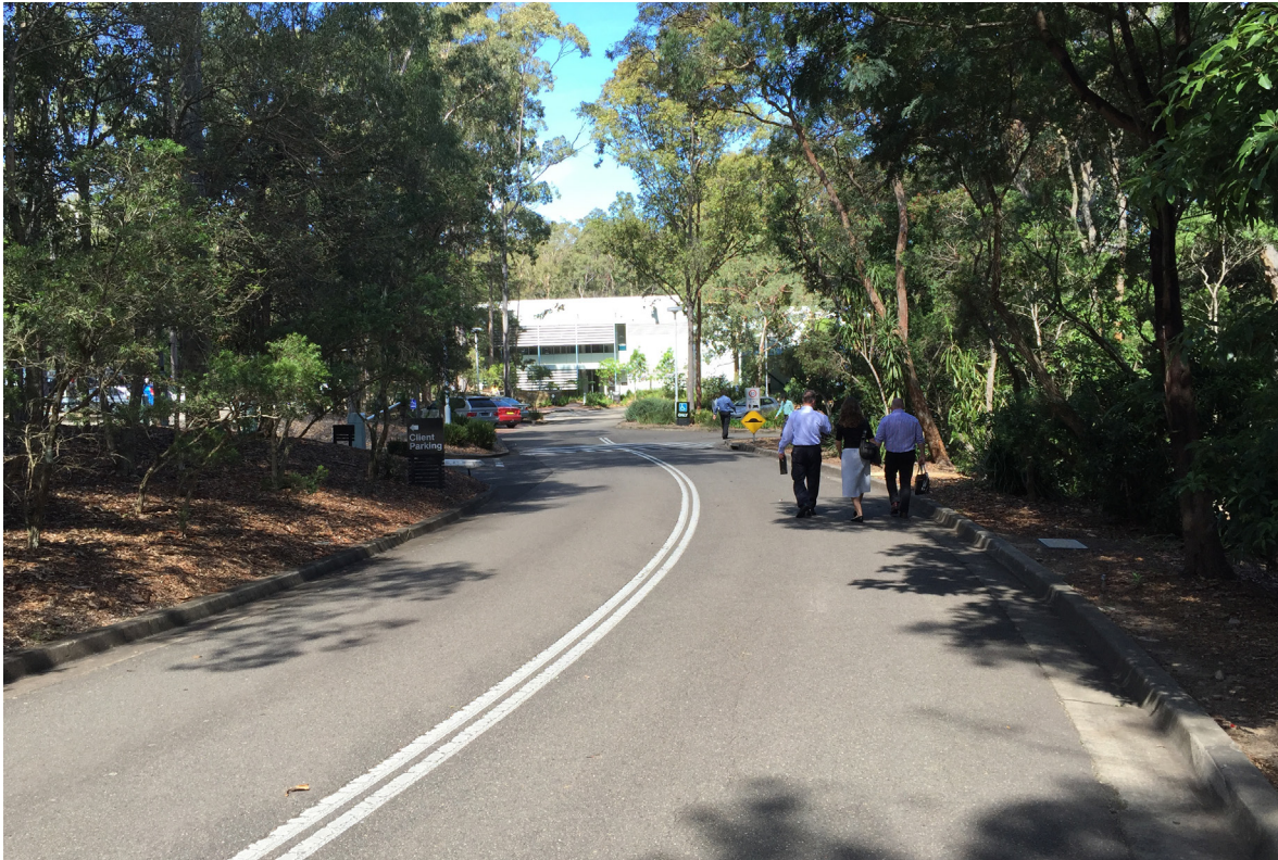
Existing Access Road (to be retained)
